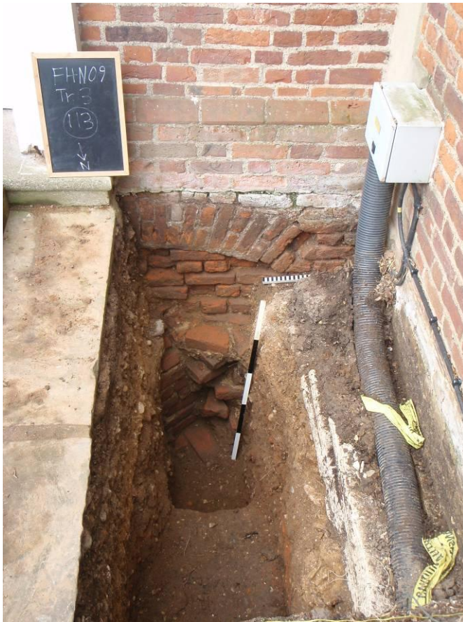
Fig. 2: The relieving arch in the original courtyard wall with the drain and reinforcing brickwork in the west trench (looking south). The path on the left leads up to the staff entrance and separates our two trenches
