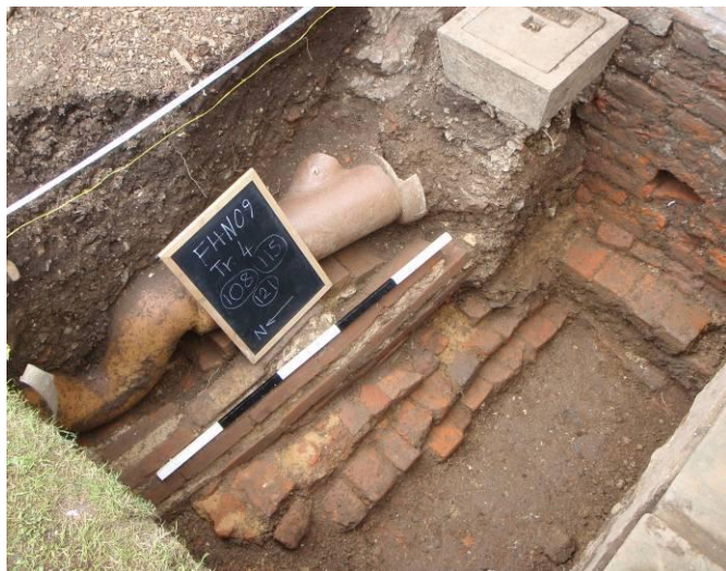
Fig. 5: The east trench looking south east with the 1660s wall's stepped foundation running up to the c. 1708 section of the facade wall of the hall (top) with its broadened base and bottom course running out of line. On the left the early nineteenth century brick built drain is still in place above the 1660s wall and above it is an ?1897 replacement pipe (the square feature is a modern lightening conductor ground block)
